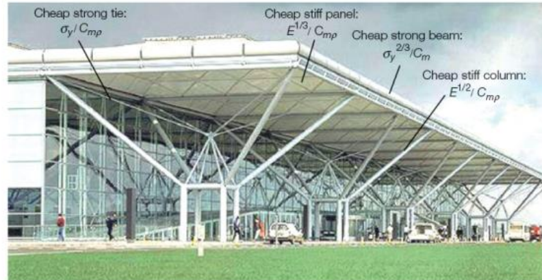
Structures with components loaded in tension, bending, torsion, and compression with material indices. (Image of Stansted Airport courtesy of Norman Foster and Partners, London.)
